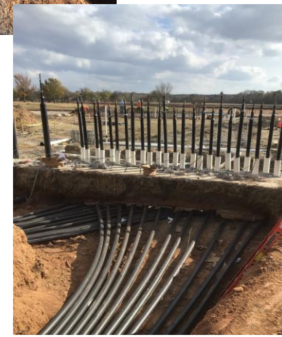
163 WELLS, - 400' DEPTH - ENHANCED GROUT
